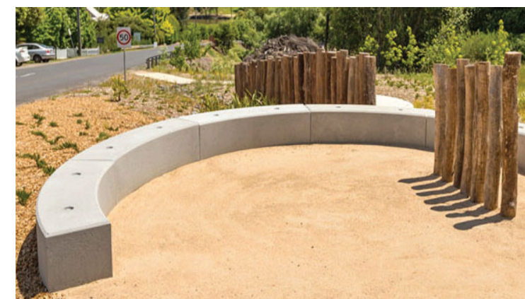
Seat Wall - Concrete
