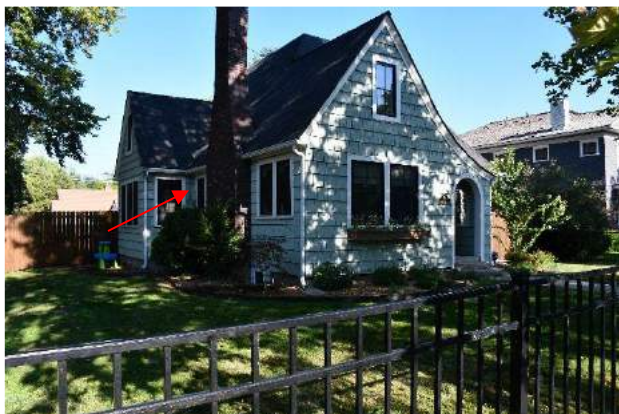
DSC_2846- Front of [REDACTED] N 19 th Street home overview. Defect in the window towards the left of the chimney.
