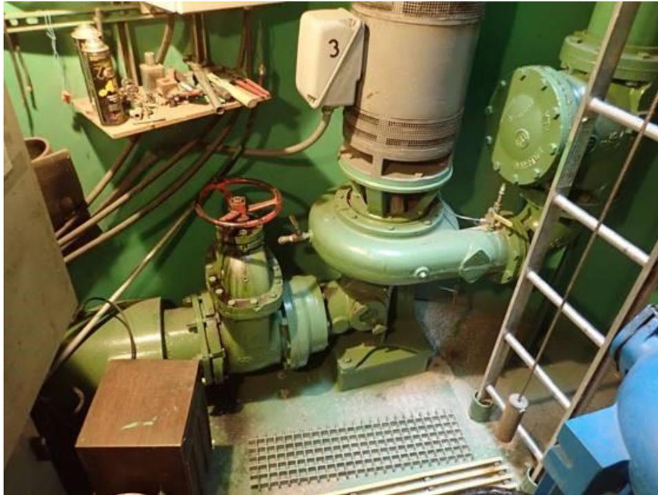
*Figure 3 - Regional Lift Station showing one of three pumps. This lift station is critical to the water renewal system and pumps over one million gallons of used water a day and has been in service for over 30 years.*
