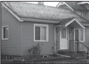
This home's replacement windows are inappropriately sized and configured. The window openings were altered and windows were changed from wood, double-hung windows to vinyl horizontal sliders, and the window frames were replaced with simpler, thinner
