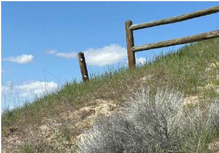
Photo 42 Plot: AA-9 4/9/2024 Fence needing repair by the plot.
