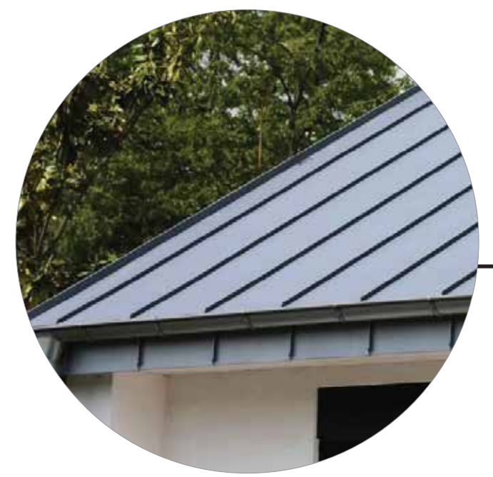
Standing Seam Metal Roofing
