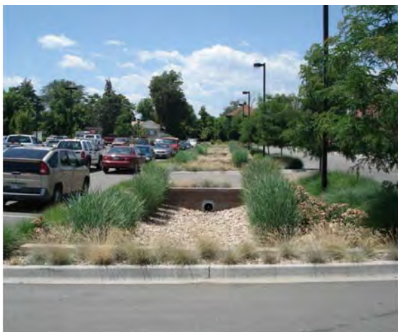
On-site stormwater improvements help reduce the amount of water in the city’s system during high precipitation while also removing pollutants.
