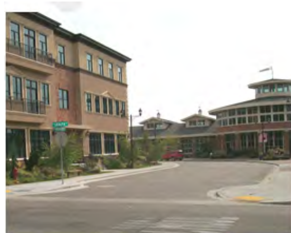
Retail and multi-family residential uses in this activity center are horizontally mixed and well integrated—both visually and physically.
