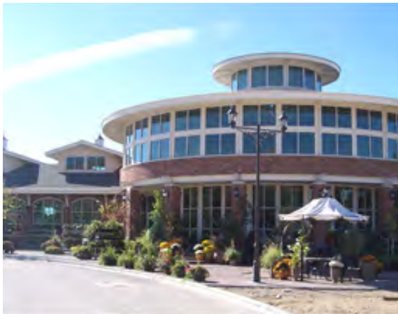
The 36th Street Garden Center received a Silver LEED certification from the U.S. Green Building Council for its sustainable design.
