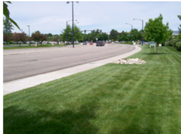
Identifiable corridors create an attractive place to shop.
