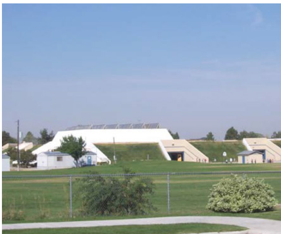
Amity Elementary School is designed with earth cover as well as solar panels.
