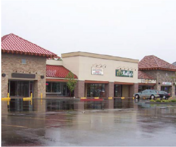
The rehabilitation of existing strip centers through façade and landscape enhancements is encouraged.
