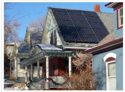
*These inappropriate collectors contrast too strongly with and overwhelm the character of the historic roof. They are also not sufficiently set back from the primary facade.*
