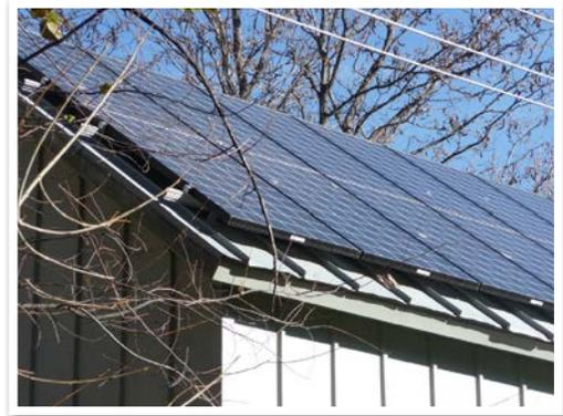
*Exposed hardware, frames and piping on solar arrays should have a matte finish and be consistent with the color scheme of the structure.*
