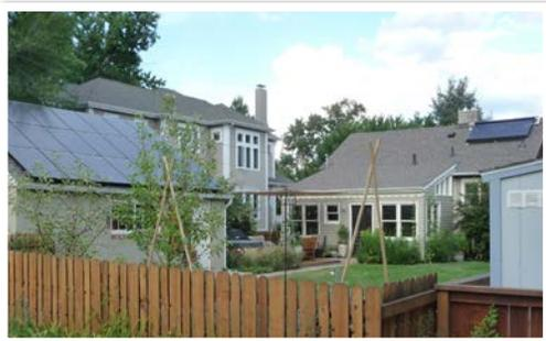
*This home uses two appropriate locations for solar collectors, on the roof of a new secondary structure, and on the rear portions of the roof on the primary structure.*
