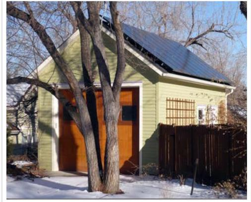
*Locating solar collectors on a secondary structure is a preferred approach. In this case, solar collector panels are located on the roof of a new garage.*
