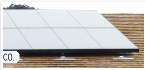
*Attach solar collectors to a historic roof in a minimally invasive and reversible manner. In this example the panels are mounted such that the original shingles are saved.*
