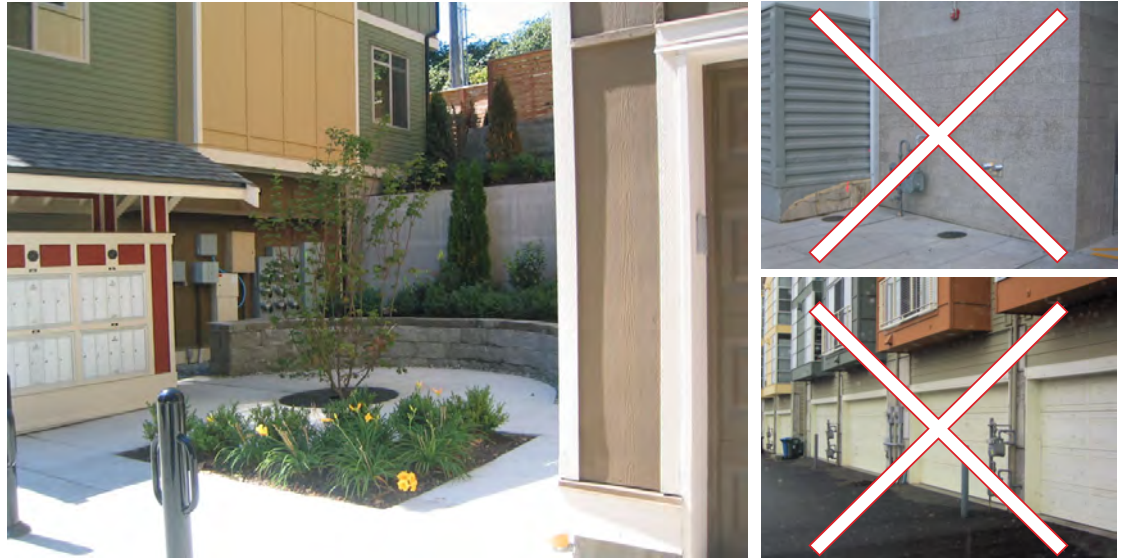
Fig. 3-18. The utility meters in the left image are accessible for functional use, but thoughtfully located and screened. Avoid exposed utility meter designs like those in the upper and lower right images, which degrade the character of the development.
