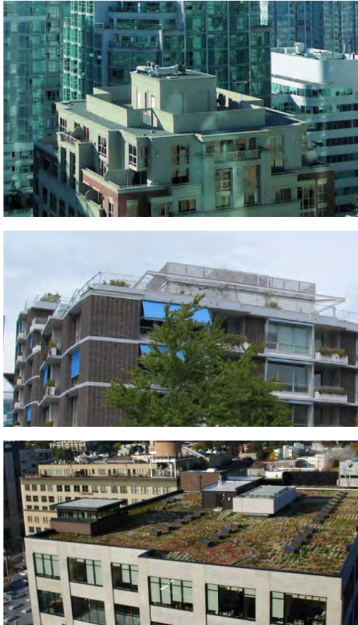
Fig. 4-37. Mechanical areas screening integrated in rooftop design.
