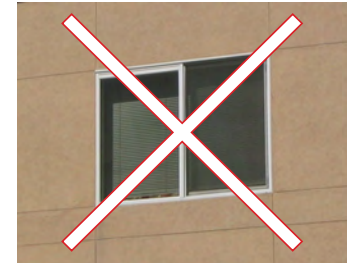
Fig. 4-46. Example of window without sufficient depth or trim.
