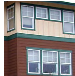
Fig. 4-45. Example of 4" contrasting trim (appropriate for buildings outside of the Downtown Core).
