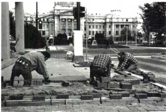
Figure 61. Handsome brick pavers similar to those at the depot being set into place for the Key Financial Center block.
