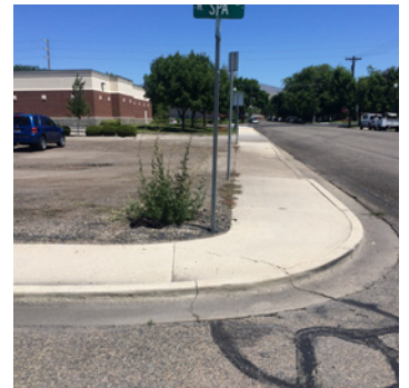
I. In the River Street area, curb cuts are unpredictable. This corner has no pedestrian facilities.
