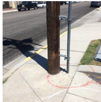
H. In the River Street area, utility poles have been placed dangerously in the center of narrow sidewalks.
