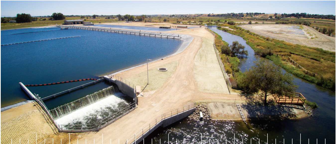
Dixie Drain Phosphorous Removal Facility near Parma
