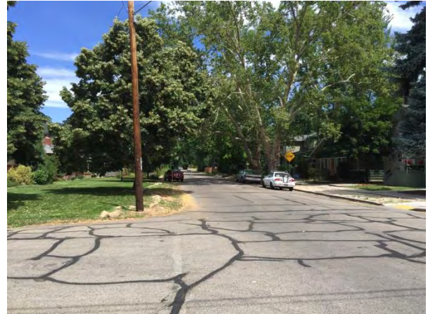
Potential Tree and Utility Pole Conflicts in Possible Sidewalk Location
