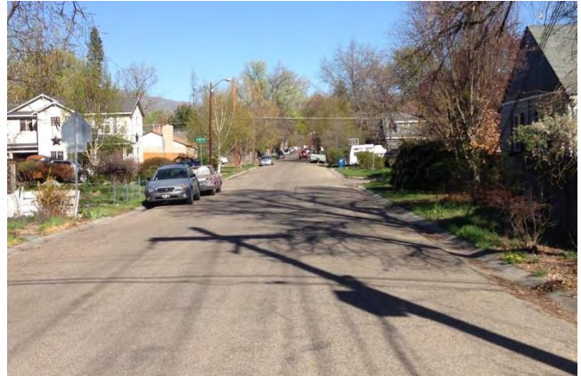
Many Local Streets Outside the North End Neighborhood Do Not Have Sidewalks
