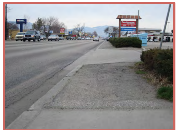
Many parts of Fairview Avenue, West Bench's busiest commercial street, have incomplete sidewalks
